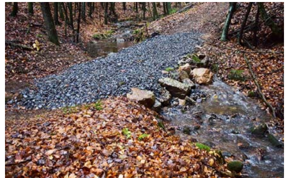
The new creek crossing.
